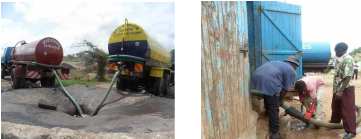
Figure 5: Private exhaustion of a pit latrine at Dagoretti Corner Nairobi at a cost of KSh 10,000
