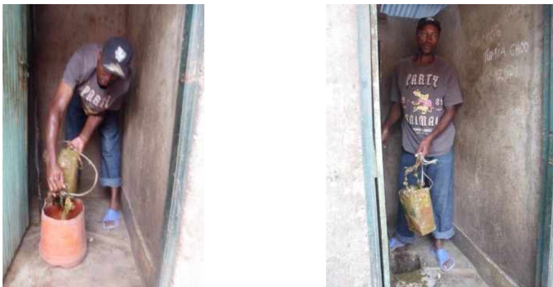
Figure 1: Emptying with a tin attached connected to a string and a bucket
